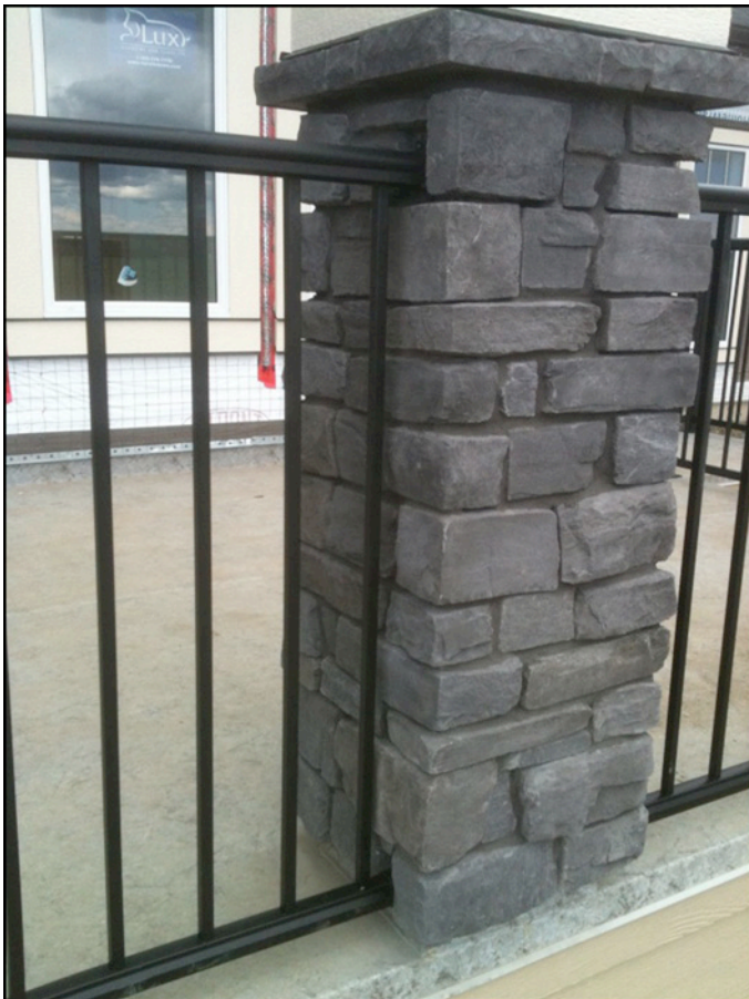
Wall Brackets Installed Prior to Rock
